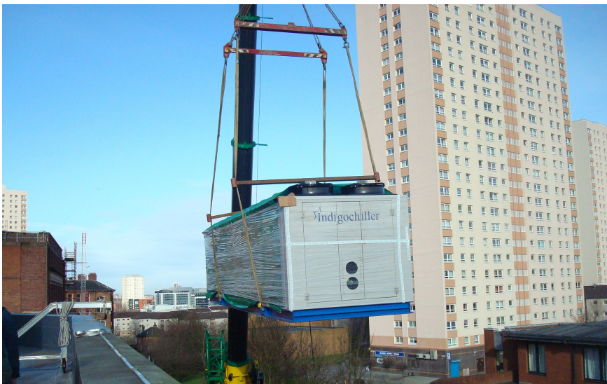
A crane lifts one of Star's Indigo chillers into position on the roof of the Curran Building of the University of Strathclyde.
